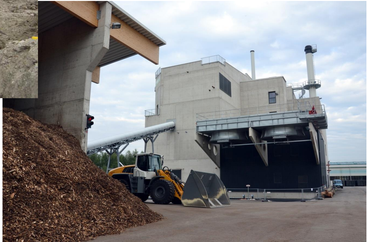
Combined Heat & Power (CHP) plant
