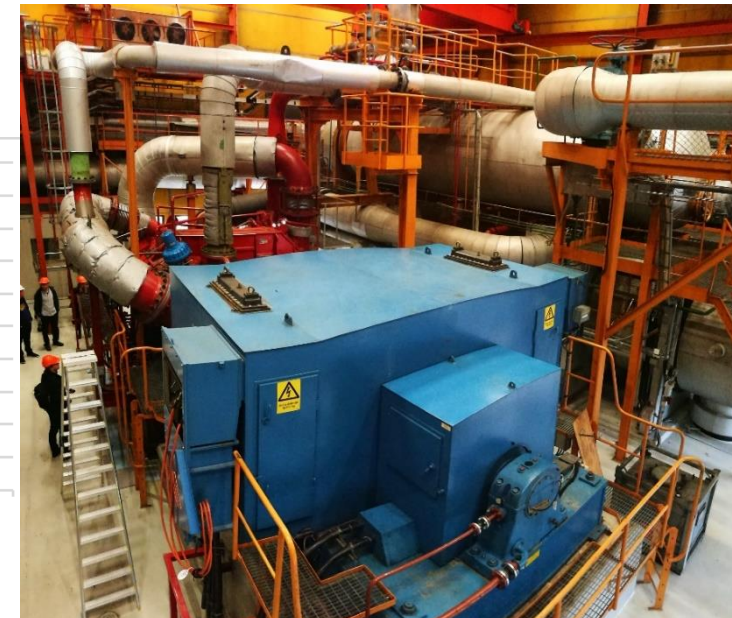
Largest Heat Pump at Rya Heat Pump Plant, Gothenburg (own photo)
