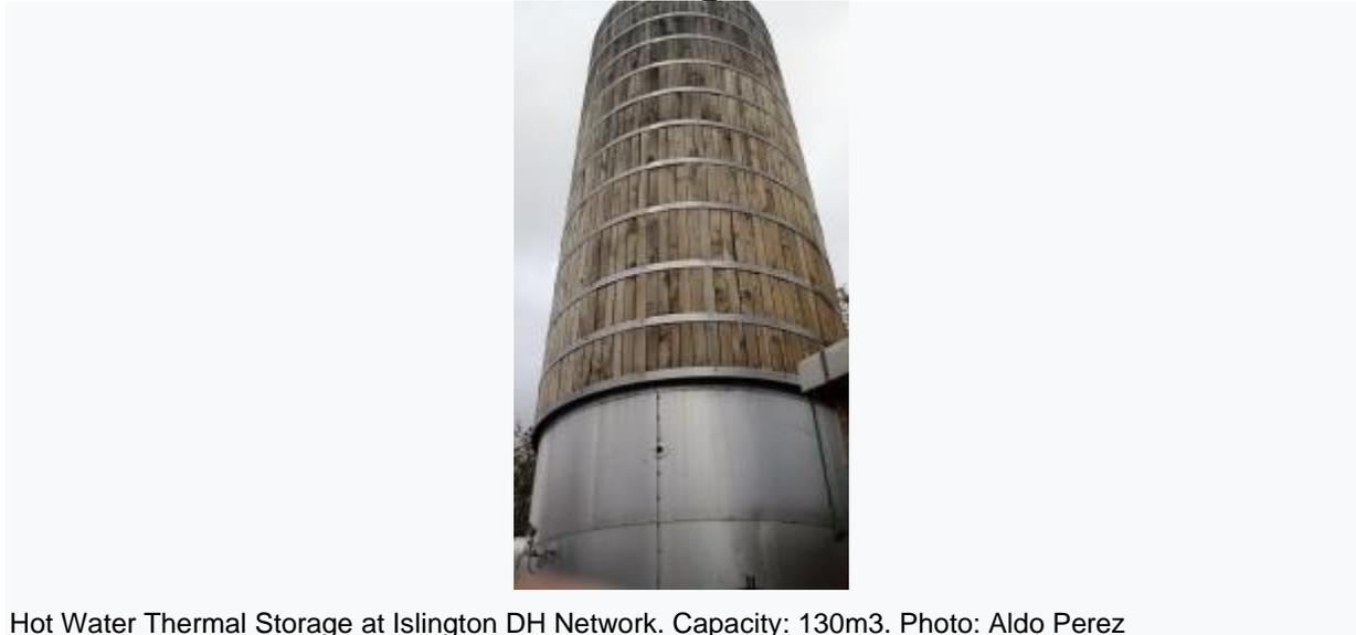
Hot Water Thermal Storage at Islington DH Network. Capacity: 130m<sup>3</sup>. Photo: Aldo Perez
